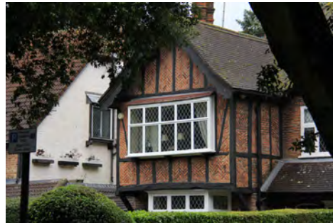
Picture 6.71 Gable end, jetty, oriel window and red brick herring bone pattern
