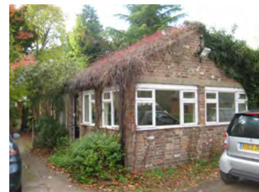
Picture 6.48 Simple single storey brick building
